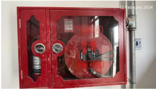
Fire hose and fire extinguisher cabinet.JPG
